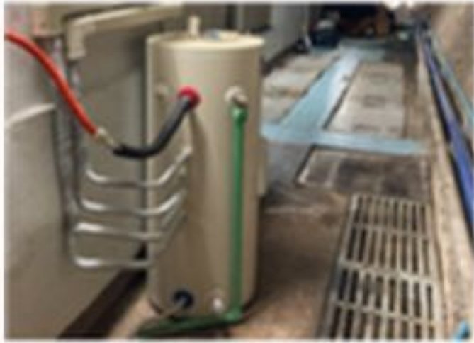
Hot water from A/C condensing unit
