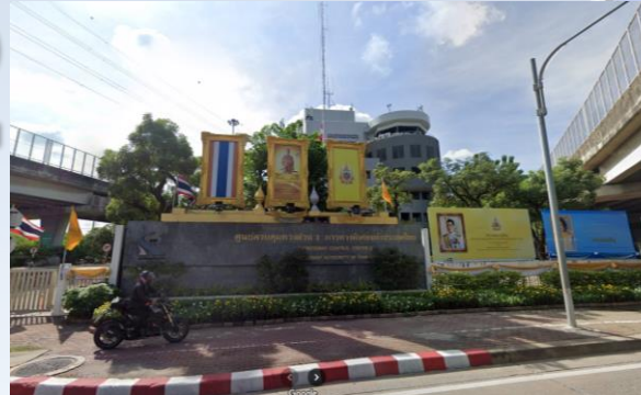
Expressway Control Center CCB1 CCB 3 CCB 4 CCB 6
