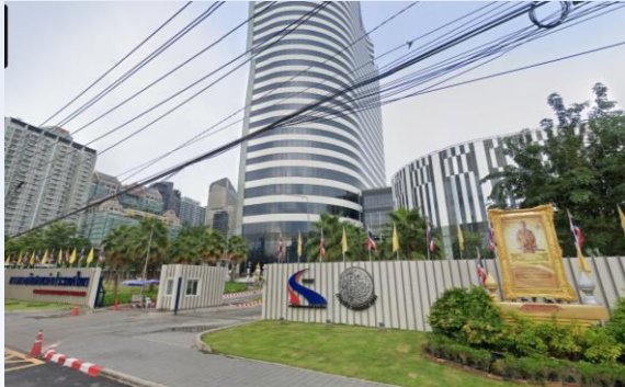
EXAT Expressway Administration Center
