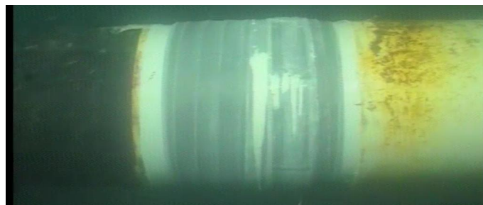
Fig. 22—Finished repair post Nautilus retrieval.
